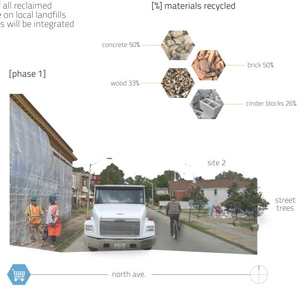
During the construction phase, buildings will be covered in plastic sheeting to reduce the amount of dust and potential harmful chemicals from entering the atmosphere.
