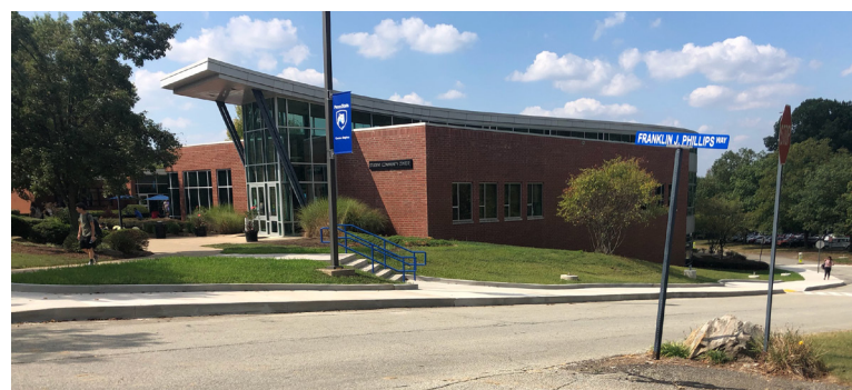
A new sidewalk along University Drive was part of summer campus renovations, as were rooms and offices in Frable.
