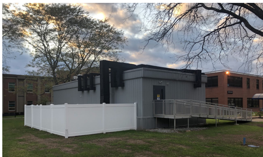
This non-descript building between Frable and Main is the Ostermeyer Lab. It will be here for two years while the Ostermeyer Building undergoes renovations.
