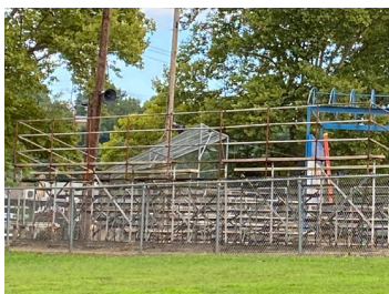
Construction equipment at Renziehausen Park
