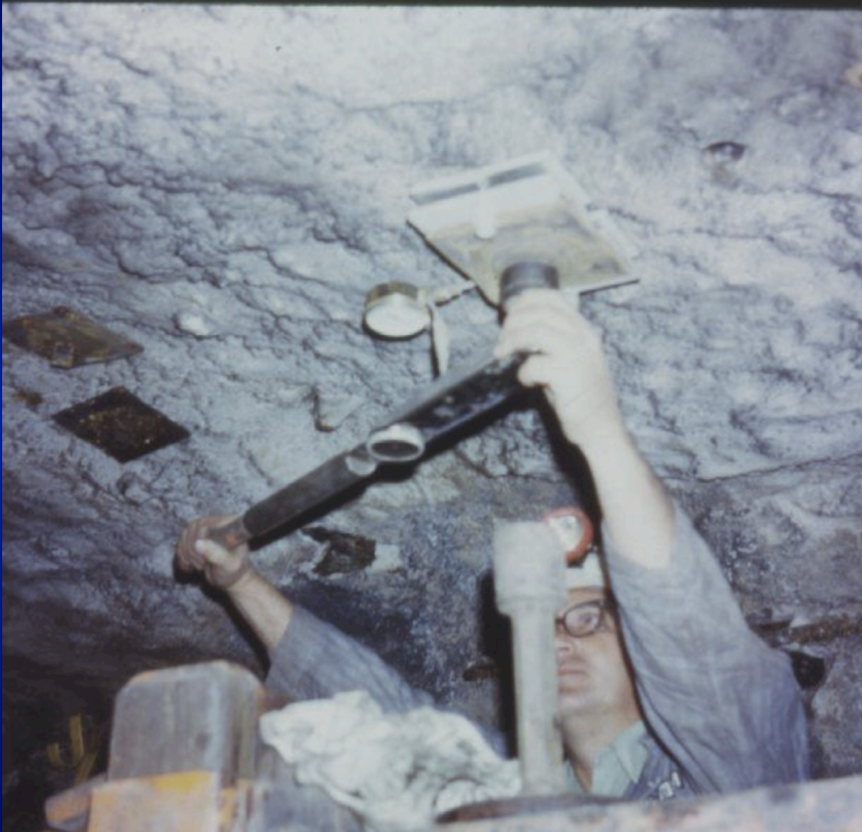
RCD Engineer Checking Installed Roof Bolt Load
