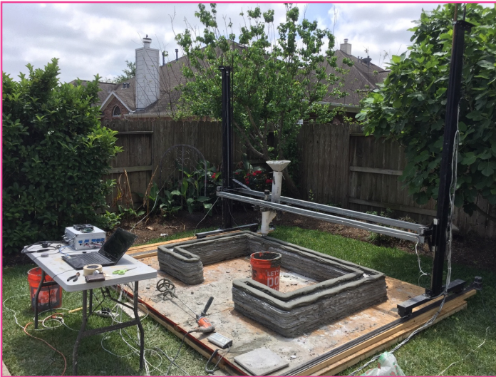
Figure 1. The tiny house during the printing process.
