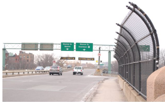
Fig. 12 – The narrow stretch of sidewalk is all that is afforded to pedestrians.
