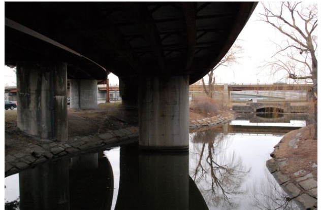
Fig. 8 – The overpass's support columns drop down into the river.
