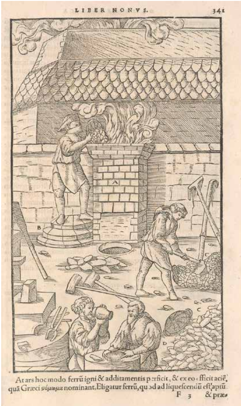
Figure 0.4. Georgius Agricola, Woodcut depicting iron smelting process, from De re metallica (1556), Book IX, p. 341. Photo: Library of Congress, Lessing J. Rosenwald Collection
